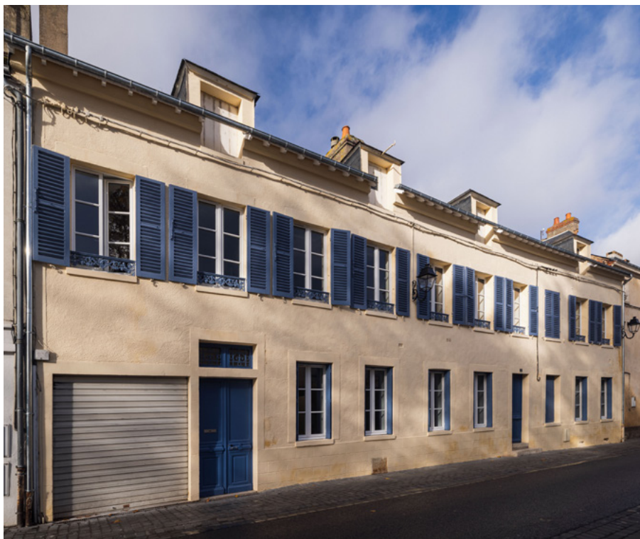
Acquisition #17 - 6, rue Pérrier 45200 Montargis
